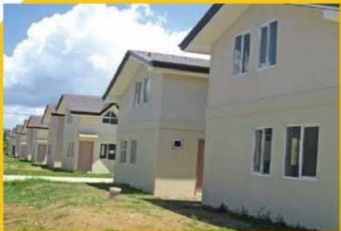
▲ Affordable houses constructed with plaswall technology.
